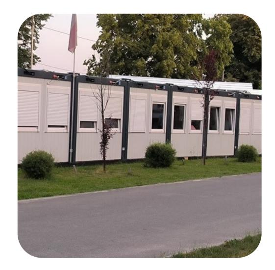
There was no air conditioning in the built modular town in Bucha. The modular structures, essentially repurposed containers, were equipped to temporarily accommodate IDPs and people who lost their homes due to hostilities. The containers are made of metal, and they get very hot at high temperatures, which makes it impossible to stay indoors.
